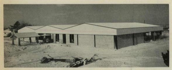
Three bays of standard metal prefab were used as the basis for the structure of the Elk's Country Club in Hamilton, Ohio, by Architects Casaccio and Loewe. Boldly projected fascia simplified joining of metal siding to the masonry walls.
