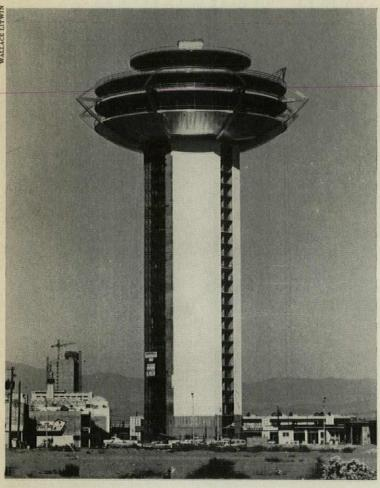
LAS VEGAS HOTEL. Soaring 300 feet out of Las Vegas' neon junk-yard, the new Landmark Hotel (above) is one of the oddest sights in a town which thrives on sensation. On five concrete pillars containing elevator shafts and stair wells sit a casino, restaurant, and entertainment areas. Cost: \$6 million. Architect: Clarence Stringer. Contractor: Caroll Constr. Co.
