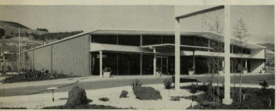
The addition of a glass end wall, overhang, and canopies to a stock 100-foot-span industrial building resulted in a straightforward but attractive design for this furniture showroom in Hayward, Calif. Owners claim they saved \$36,000 by using pre-engineered construction.
