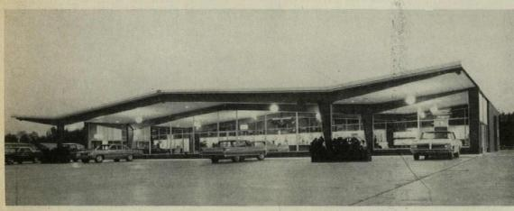
Airy automobile showroom in Bogalusa, La., was designed by Architect John Mykolyk, using 80-foot span with 20-foot cantilevers. First 24-foot bay was left open for outdoor sales. Building was completed by the contractor in only 90 days.
