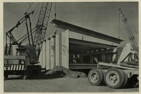
Fourteen prestressed single Tee beams form the roof; the same number are used for the floor. Roof Tees are 8' wide; range from 88.2' to 30' in length. Floor Tees are 73' long, 8' wide, 3' deep. The precast supporting columns are 34' high, 3' deep, 8" thick.
