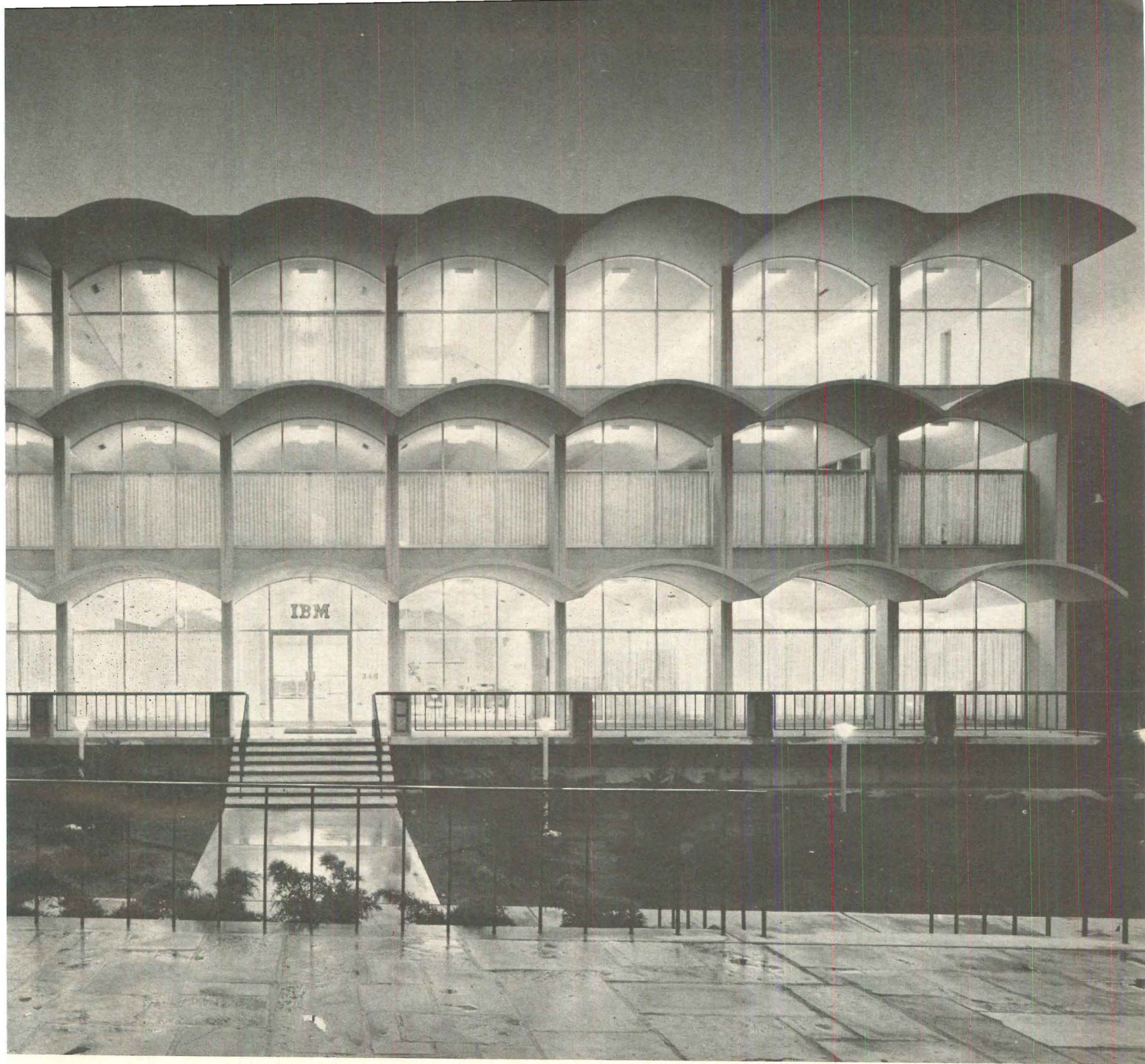
structural shells on bright display. The site drops off, so the building sits on a flared platform with a sunken garden between it and the street.
