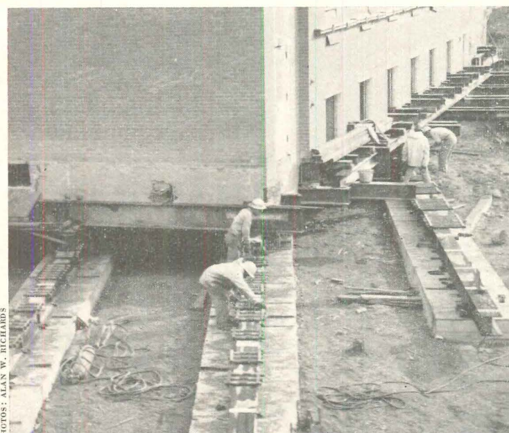
Hydraulic jacks (above) moved building along on rollers shown below
