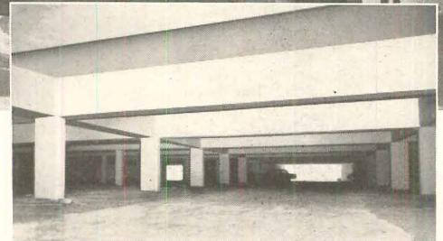
Post-tensioned beams used in underground parking garage.
