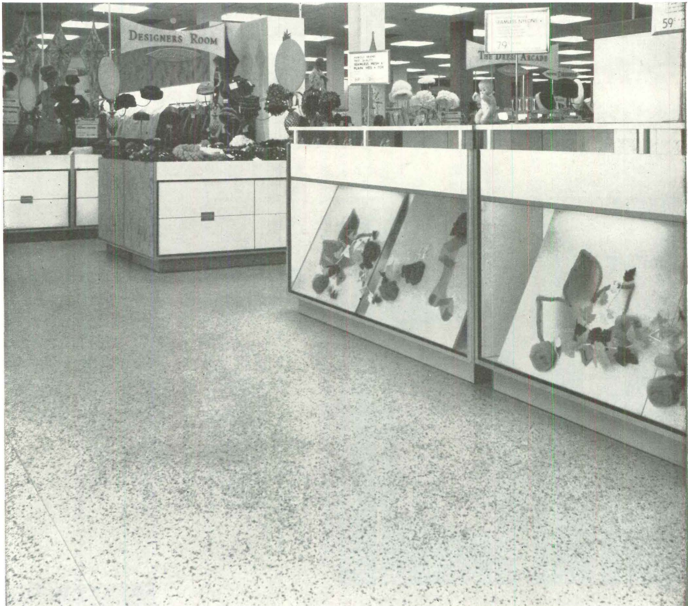
Terrazzo flooring made with ATLAS WHITE cement at S. Klein's Department Store, Commack, N.Y. Architect: A. H. Salkowitz, Jamaica, N. Y. Contractor: Jules Schneider, Inc., Hempstead, N. Y. Terrazzo Contractor: Seaboard Tile & Terrazzo Co., Farmingdale, N. Y.
