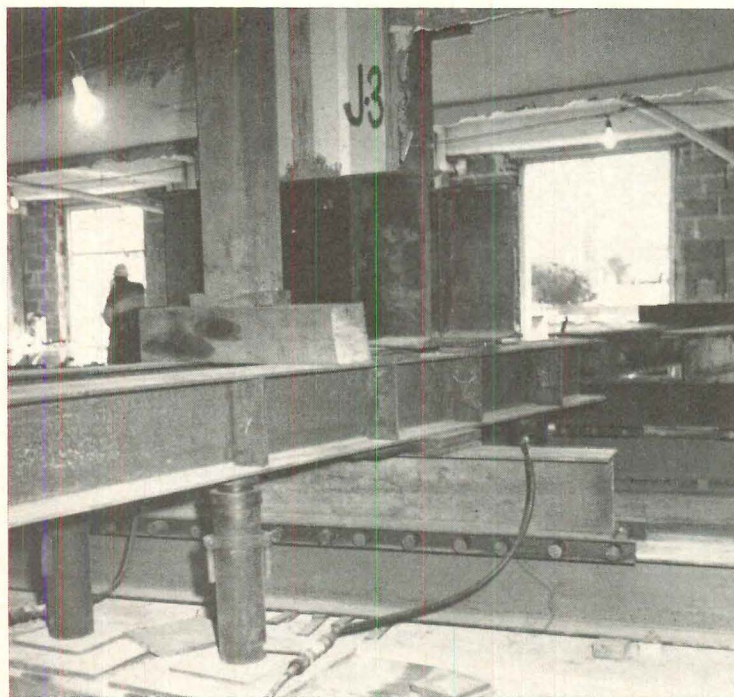
The five layers of steel required to shift structure are seen above
