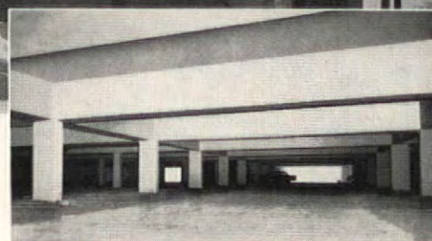
Post-tensioned beams used in underground parking garage.
