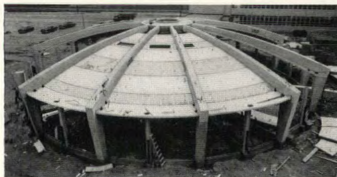
44-foot, 12-ton beams, precast with "Incor" 24-hour Cement, rest on cast-in-place center core and on 13-foot precast columns on the outside.
