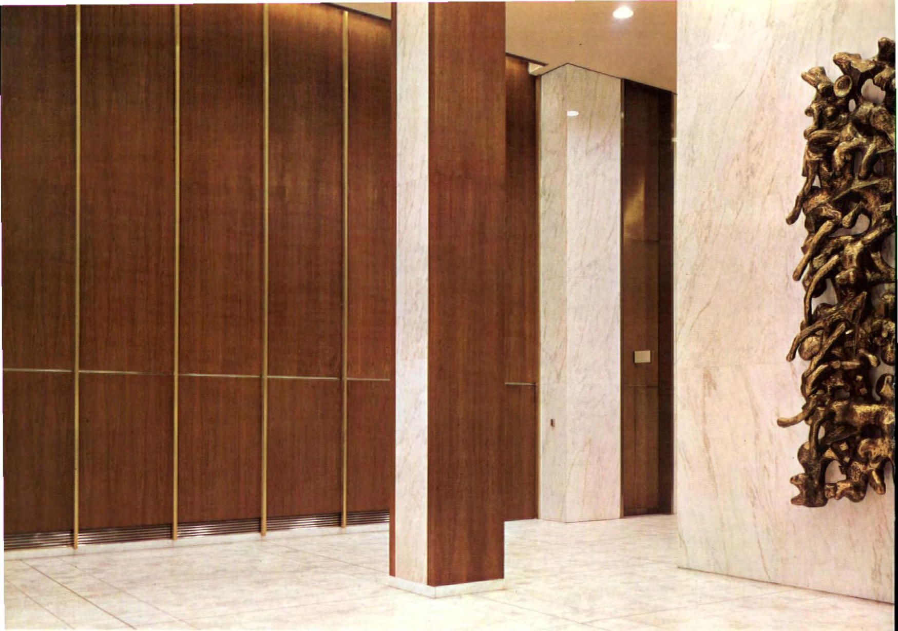
Weldwood Algoma Architectural-Grade Custom-Made plain sliced cherry paneling in lobby of Union Tank Bldg., Chicago, Ill. Top panels are 16' 3" high. The 7' panels below are end-matched with top panels. All panels are 5-ply with lumber core, were completely premachined and prefinished at our Algoma plant. Bldg. owner: National Properties, Inc. Architect: A. Epstein and Sons, Inc., Chicago, Ill. General Contractor: George A. Fuller Co. Installer: Peterson Co., Chicago.
