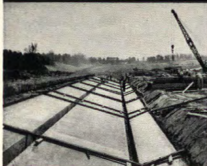
This is the concrete bed on which roof units are cast. Roof units as well as all the other precast structural units are 3,000 p.s.i. lightweight concrete.
