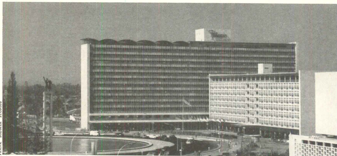
INDONESIAN HOTEL (left). Completed in time for the Asian Games in Djakarta last year, this 14-story hotel designed by Architect Abel Sorensen is the biggest in southeast Asia. The 450 rooms are also intended to open up Djakarta to foreign businessmen, who previously had no place to stay. Bright-colored sun breakers in enameled steel shade balconies on the main building, while an eight-story wing has aluminum brise-soleils to reflect sun and counteract an east-west exposure. An Olympic-sized swimming pool, a 1,200-seat auditorium, and a nightclub are included in the Western-style accommodations.
