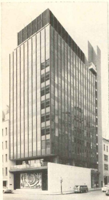
MANHATTAN CENTER. This bronze- and glass-sheathed office building, designed by Architect William Lescaze, stands directly across from the United Nations and houses various U.N.-related church agencies. The structure is of reinforced concrete, and has outdoor terraces on the second and 12th floors. For the street-floor chapel, Henry Lee Willet designed a mural-like window of faceted chunks of glass set into a 13 by 25 foot sculptured metal wall. The $3 million Center was built under the auspices of the Methodist Church and is under the direction of the Department of International Affairs of the National Council of Churches. Engineers: Greenhut & Taffel (structural), R.L. Stinard & Associates (mechanical, electrical). General contractor: Diesel Construction Co., Inc.
