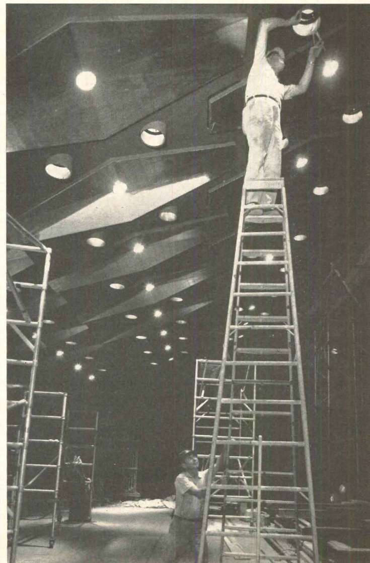
Above: the hall during tuning week, with glass-fiber batts simulating audience absorption. Below: the "clouds" raised and the gaps filled in.
