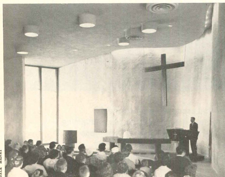
TEXAS CHURCH. The massive walls of the St. Stephen Methodist Church, in Mesquite, Texas result from an unusual and economical new construction technique: they are made of concrete block laid without mortar, then covered on both sides with a cement-base spray coat. The free-form church, which resembles a sort of prairie
