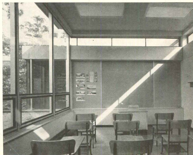
Offsetting classroom roofs, above, permitted clerestories shown below
