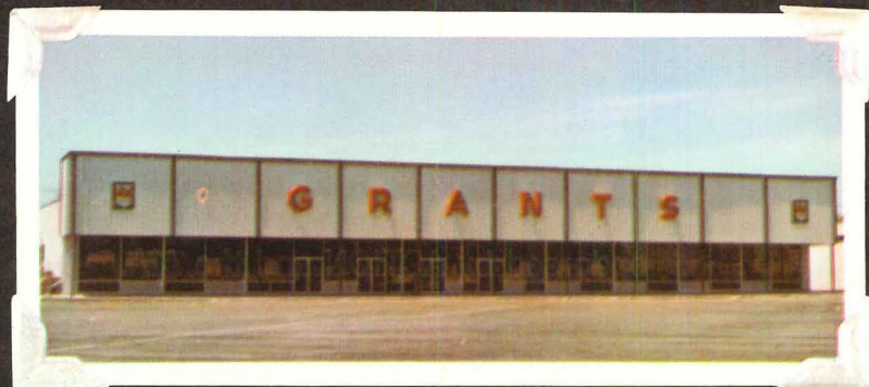
W. T. Grant Company store, Port Jefferson, Long Island, N. Y. Architect; Frederick Saphier, New York City. General Contractor; Reliable Construction Co., Bronx, N. Y.
