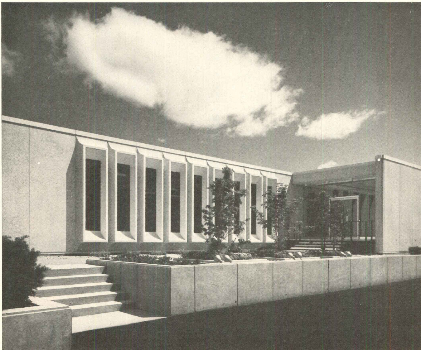
IBM Building, Kalamazoo, Michigan. Architect: Ezra Gordon, Jack M. Levin & Associates, Chicago, Illinois. Contractor: Miller-Davis Company, Kalamazoo, Michigan. Concrete Panel Manufacturer: Crest/Schokbeton Concrete, Inc., Lemont, Illinois.
