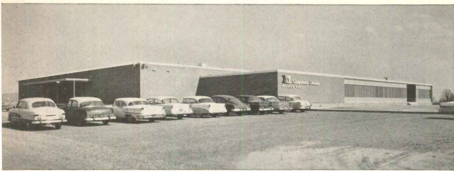
A FACTORY IN VIRGINIA —I. T. T. Components Div. Plant, Roanoke. Architect: John D. Latimer. General Contractor: C. M. Guest & Sons. Masonry Contractor: Saunders & Divers. Lightweight Concrete Block: Webster Brick Co., Inc. Ready-mixed Concrete: Concrete Ready Mixed Corp. and Roanoke Ready Mix Concrete.
