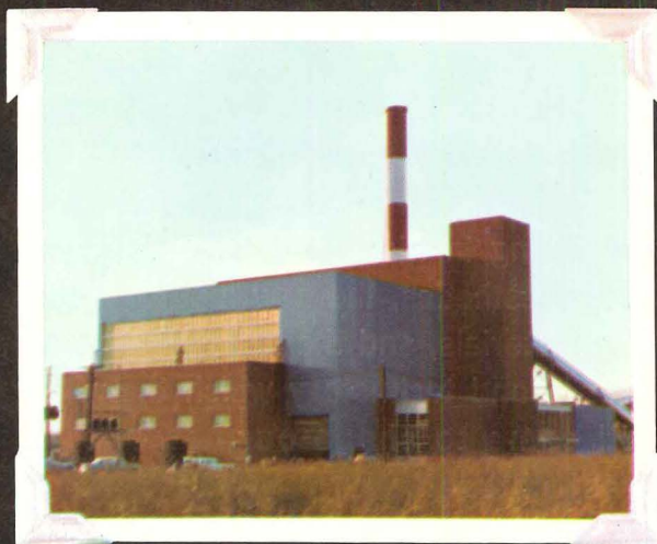
McKee Run Generating Station, City of Dover, Delaware. General Contractor; Somers Construction Co., Bala Cynwyd, Pa.
