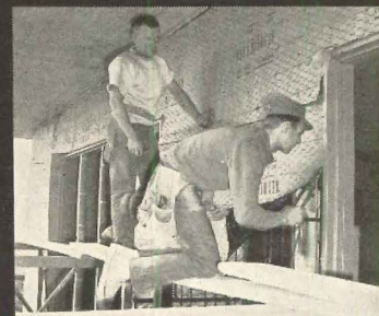
Then Keymesh Paperbacked lath is applied.
