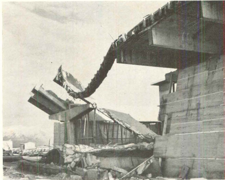
Shocks buckled the roof of a partially completed, prestressed concrete building
