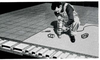
Cellular steel subfloors provide invisible electrical flexibility, with outlets where you want them, anytime. Larger cells function as secondary supply ducts in the air conditioning system.
