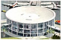
Resilient Barrett urethane insulation follows the contours of the "dish" roof on the Carson's O'Hare Airport restaurant in Chicago. Architect: C. F. Murphy Associates.
