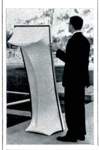
looks: this bench is made of glassfiber-reinforced plastic and weighs only 50 pounds, a lightweight as outdoor seating goes. Compound curves underneath strengthen the bench so that it won't tip over if a single person sits on one end. Douglas Deeds, who designed it for Architectural Pottery, curved the seat for comfort and dipped the ends a bit for rain runoff. For fixed installations in concrete, the manufacturer will supply studs on the legs at no additional cost.
