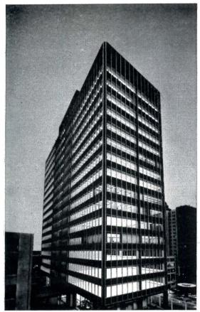
Parallel-O-Grey plate glass was used to glaze the Norton Building, Seattle, Wash. Architects: Bindon & Wright. Associate Architects: Skidmore, Owings & Merrill.
