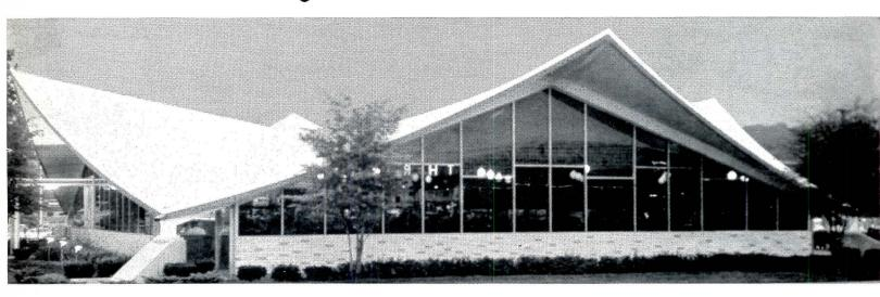
The owners of Frisch's Restaurant, Cincinnati, wanted a striking structure, a square open floor plan, and moderate cost. These requirements were fully satisfied with an economical thin-shell hyperbolic paraboloid roof of steel deck.
