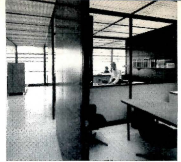
Partitions plug into ceiling module
