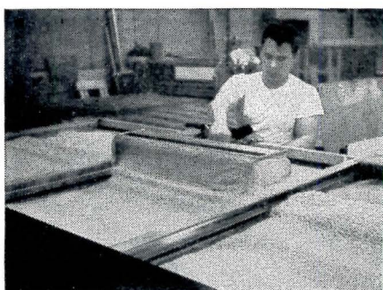
Moisture-resistant urethane eliminates need for separate vapor barriers in complex louver shapes.
