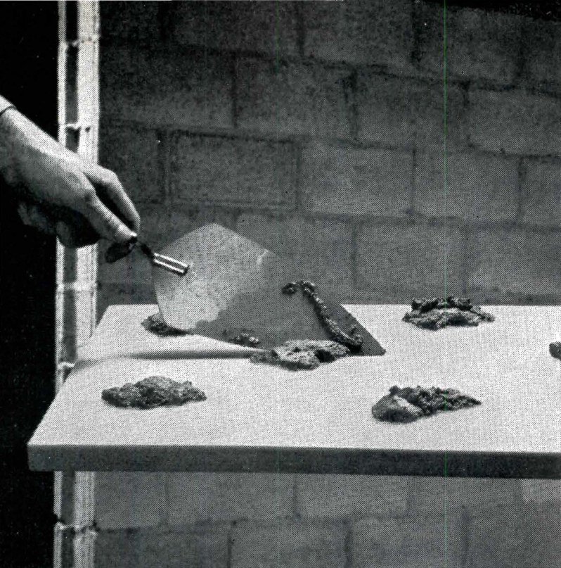
3. Spot-apply Styrotac® bonding adhesive.
