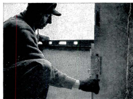
Panels are bolted in place at the job site. No fussy handling is required to avoid damage.
