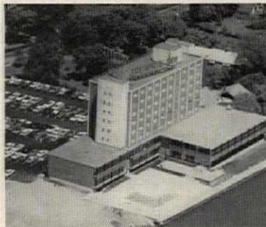
New Treadway Inn, Niagara Falls, New York. George E. Yurchison, Architect. An all-electric building.
