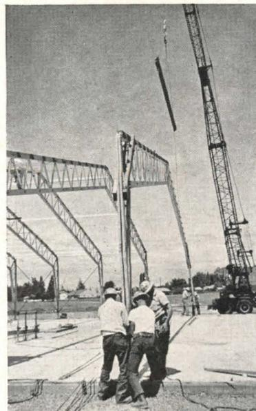
TRUS JOIST's perfect blend of wood and steel offers unique design freedom with economy. That blend provides much more too... light weight for easy erection and for savings in foundations, footings and bearing walls ... available top and bottom chords for the attachment of low cost roofing, ceiling and flooring materials... open webs for duct work and wiring... minimal deflection in spans up to 100 feet.
