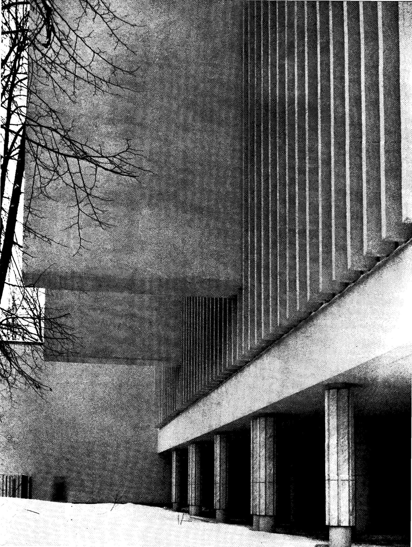
THE STRUCTURE of the student club is concrete, the walls plaster-covered brick painted white. Along the north side (left) run vertical precast concrete baffles, and the columns here are, in typical Aalto fashion, wrapped in marble strips. The building's main halls are windowless: behind the baffles is a lofty gallery (right), glazed on both sides, carrying a series of ceremonial stairways.
