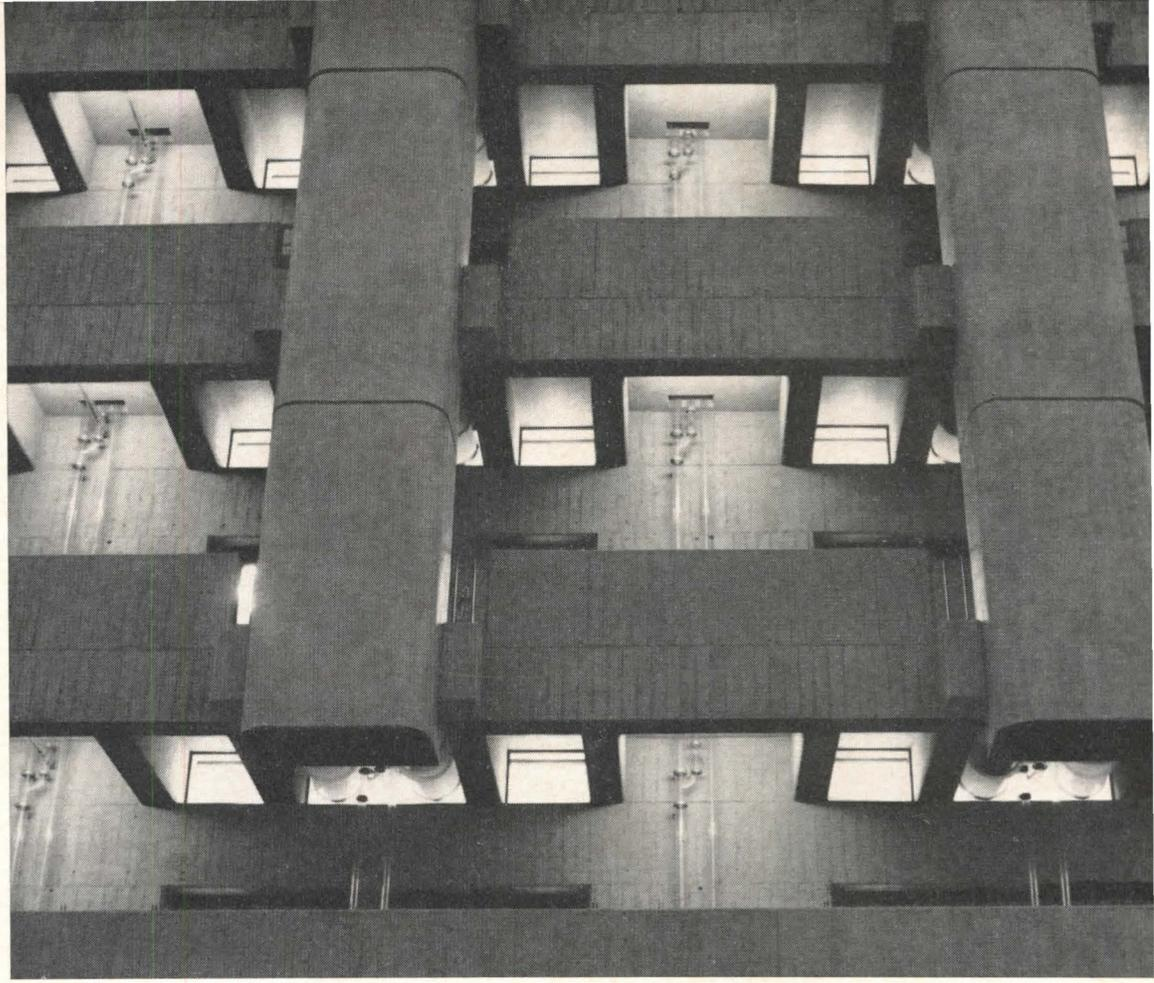
**An exposed slab, with deep beams as ribs, provides the required ceiling height.**
