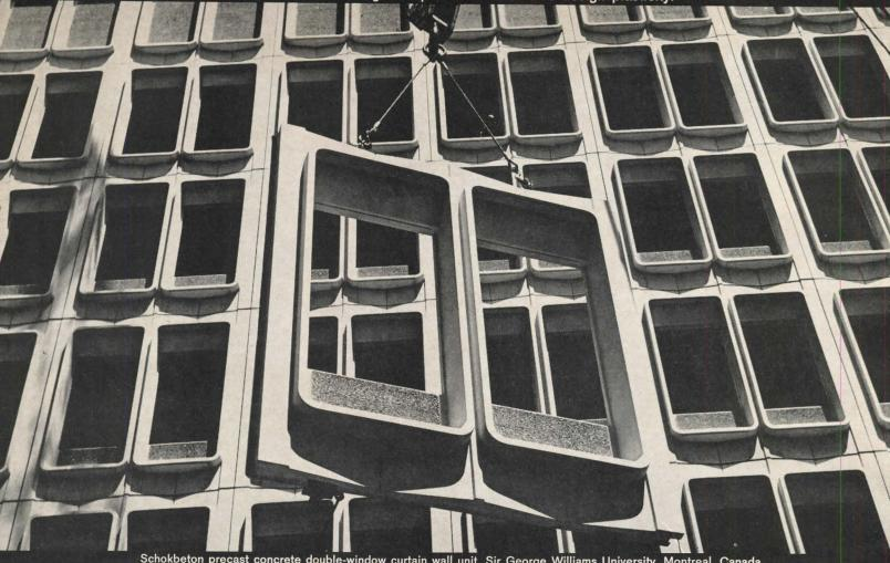
Schokbeton precast concrete double-window curtain wall unit, Sir George Williams University, Montreal, Canada Architect: Ross, Fish, Duchesnes & Barrett. Schokbeton by Schokbeton Quebec, Inc.
