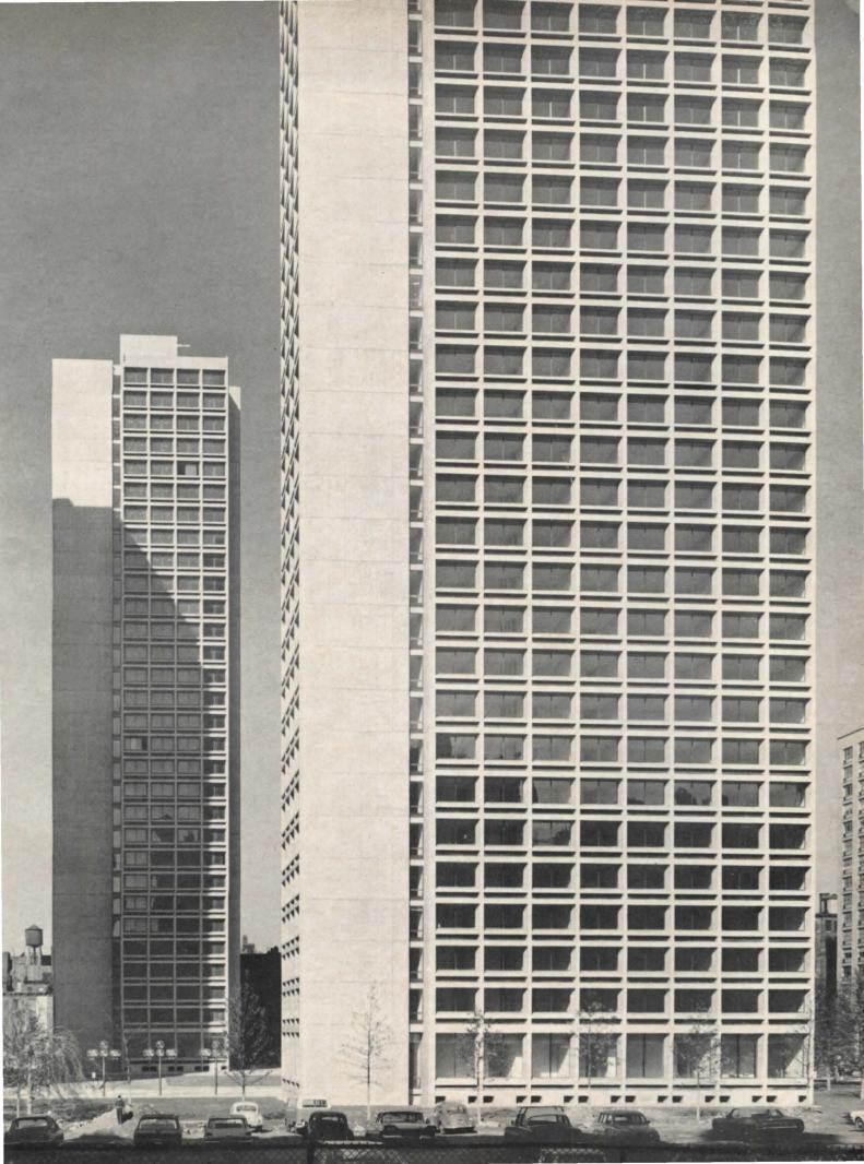
The regular grid of the exteriors was entirely poured in place. Columns and spandrels were cast in T-shaped glass fiber forms, one set per tower, with backup plates creating recesses in the columns for steam risers. The sills were cast later, in a separate operation.
