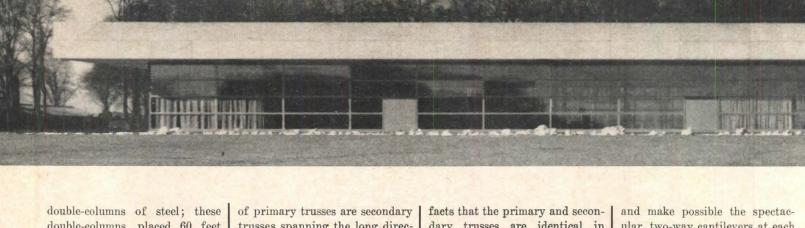
double-columns, placed 60 feet on centers, carry primary trusses in the short direction of the roof; they have a 120-foot clear span and they cantilever another 30 feet or so beyond the columns at each end.
