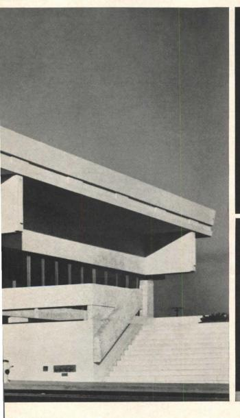
All elements of the Ventura Savings and Loan Association building, except the precast, posttensioned waffle ceiling, were job placed concrete. Interior concrete is natural color and texture. Hand railings are bush-hammered white concrete.
