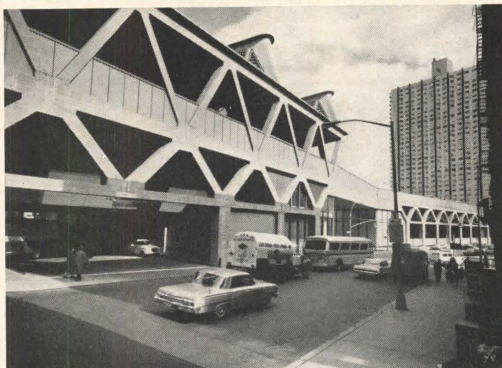
Another contrast marks the terminal's encounter with the city. At its Broadway entrance (above), the fundamental strength of the structure is negated in terms of both shapes and materials. But it emerges clearly on the side streets (below), where Nervi's angular framework carries on its intended dialogue with the lattice towers of the bridge.
