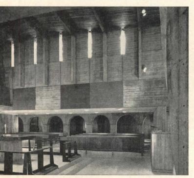
Inside walls are also exposed concrete. 1 x 6 board forms were used, and the concrete surface was left unfinished.
