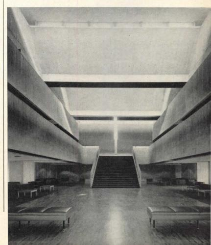
The lofty ceiling of the Student Union (photo and section left) is made up of a series of V-beams that are enclosed by light monitors above the roof (top right). The ceiling rises above an interior well containing two balconied levels overlooking the ballroom (section and photo right).
