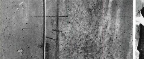
**BEFORE** 1. Concrete wall showing imperfections, varying gradations of color, honeycombing and protruding tie rods.
