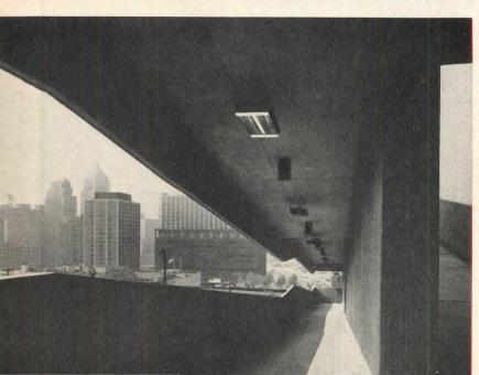
Concrete, glass, and oak (in the form of access panels for window washing) compose the facades on the front (opposite) and rear. On the sides are great scissor ramps structurally independent of the building (left top and center). A wide balcony off the sixth-floor faculty area (left) doubles as a sunshade for the floors below.
