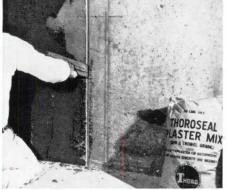
4. Trowel application of THOROSEAL PLASTER MIX-PLUS-ACRYL 60\* (one part to three parts water) is being applied to concrete surface filling all voids.
