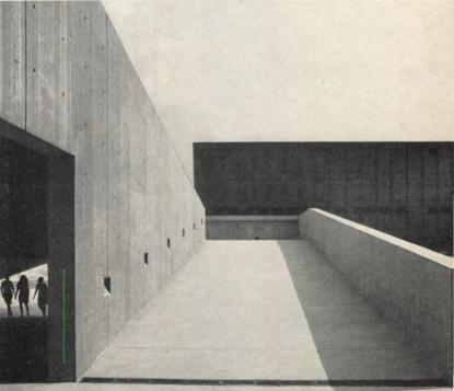
Entrance to Duquesne University's new Student Union is via a massive concrete ramp that cantilevers 28 ft. from its base (top right and detail at left). The building is the first to be completed under a master plan for redevelopment of the campus (center right). Across from the Student Union is the nearly completed Science Center (right) designed by Mies van der Rohe.
