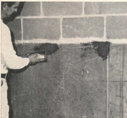
3. THORITE quicksetting, nonshrink, nonstaining patching mortar, is being forced into holes. Before doing this, workmen applied a "slush coat" of THORITE.
