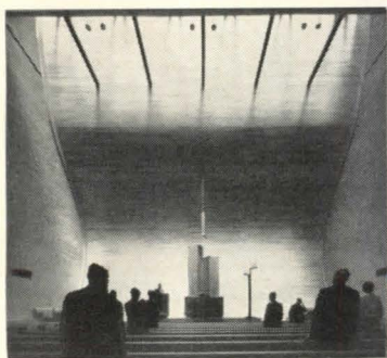
Left and above: interior of sanctuary, showing space formed by concrete shells. Front wall shell is finished inside with horizontal birch slats; rear wall shell is plastered. Space frame skylight is concealed from view of congregation so as to heighten dramatic effect. Section and plans (far right) explain the organization of the principal spaces. Basement plans (with social and conference rooms) are not shown here.
