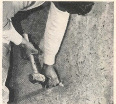
2. Workman removes loose concrete and cuts back tie rods too close to surface. Area will be thoroughly cleaned with water or forced air before patching.
