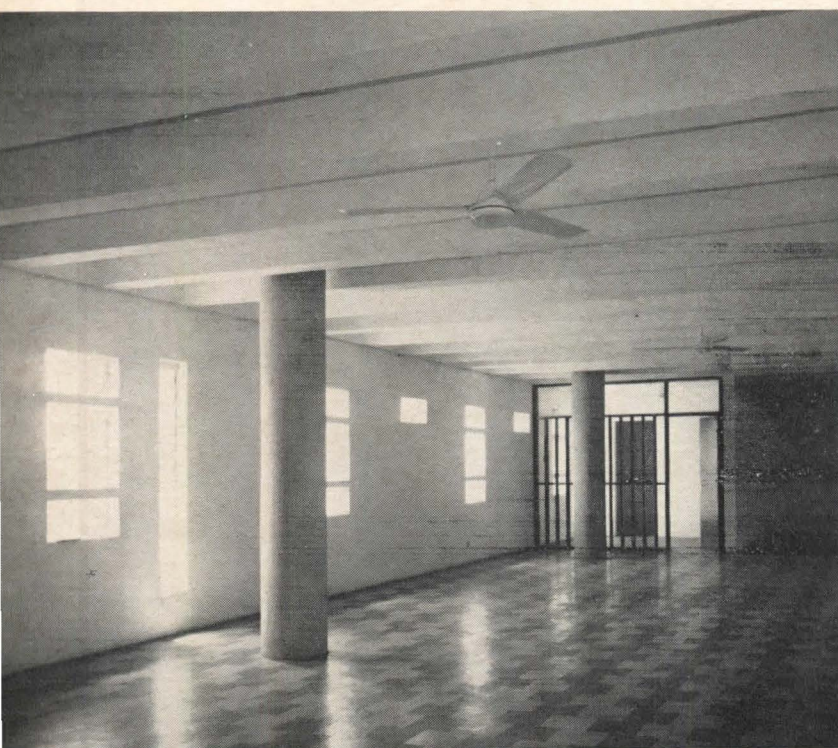
Top left: one of two open courts that separate the four elements of the library. Wall at right is part of children's library unit. Bottom left: workroom for library staff, before furniture was installed. Right: walls are stuccoed concrete block. Special blocks were used for window frames.
