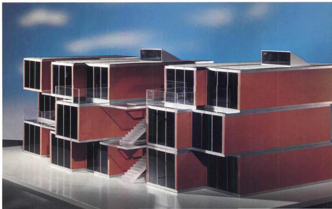
Steel frame used for bottom and middle units permits stacking three or four high.
