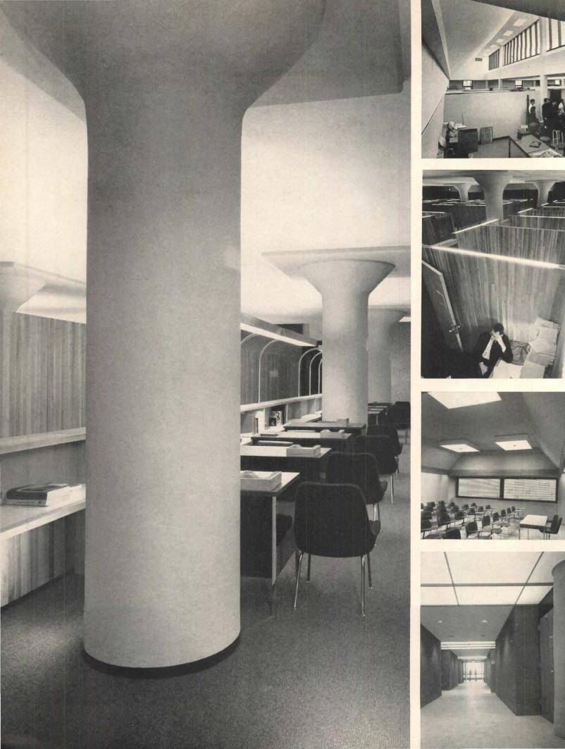
The interiors have been planned around massive columns and slabs The eight floors of the factory structure have been converted to "generalized" teaching and office space. Since it was virtually impossible to cut through the old 9½-in. floor slabs (and existing openings in them were negligible), elevators and stairs to serve these spaces were added outside of the original structure, as were toilets and fan rooms, which require utility risers.
