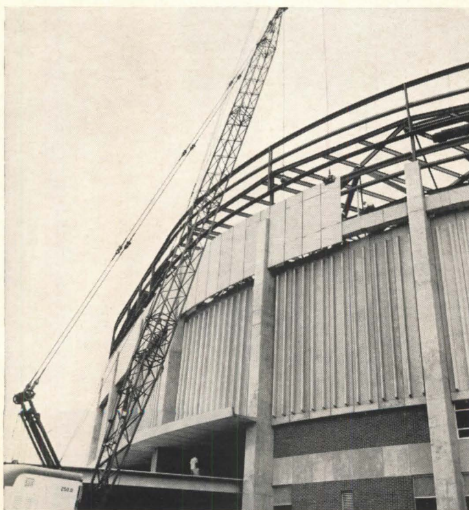
280 large precast, prestressed double T panels provide the ribbed effect of the upper walls of the new auditorium. Each measures 30' high x 48" wide. Smooth surface precast panels form the top section of the wall. A major portion of cast-in-place concrete for the structural system was pumped into the forms.
