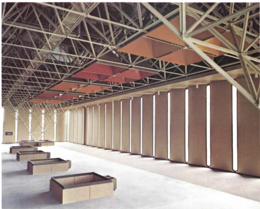
The Bethlehem Mayari R panels are constructed with painted sheet steel panels on the inside.
