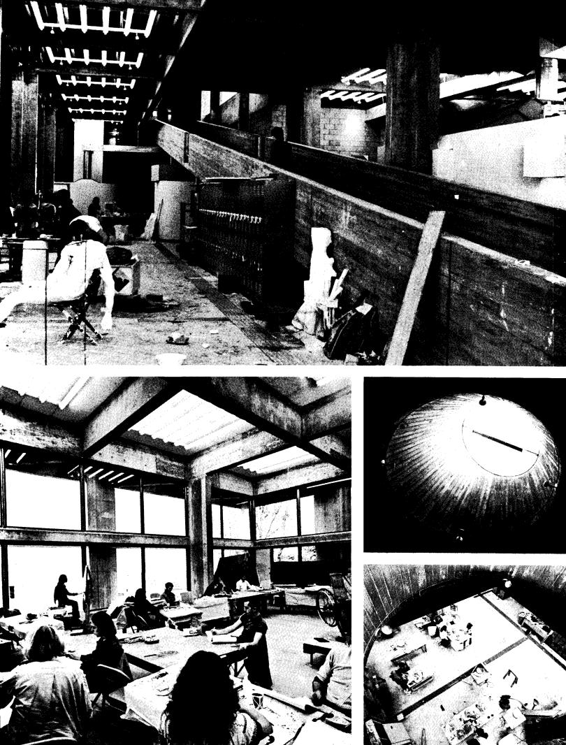
top, its untreated, unsurfaced concrete depends upon post-tensioning to prevent moisture penetration. So far it has worked, a neat way to save the cost of waterproof membrane and a separate wearing surface. Clay's concrete echos the texture of the 1927 building, but remains gray against the ochre of the old work.
