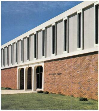
Hollow Corspan panels provide a finished outside/inside wall
