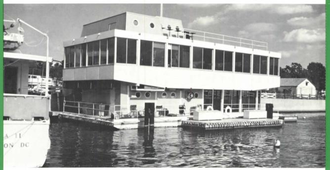
The Gangplank Restaurant in Washington, D.C., is a two-story structure atop a floating barge.
