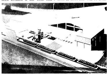
ferred to a loading dock where a mechanical lift will grab the bales and place them in waiting railroad cars for eventual transport to landfill sites. This entire automated system will be operated by a single person in a glass-enclosed control tower high above the scene.
