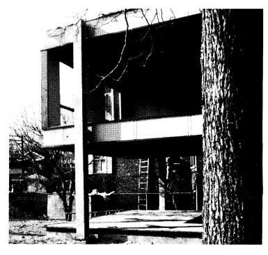
—they just lift the panel, place the lower edge in the floor channel and tilt the top into place. The seams are all waterproofed (the contractor has repeatedly sprayed water on the building to test the waterproofing).
