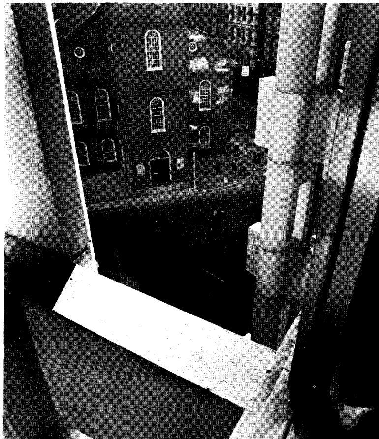
At the Boston Five Cents Savings Bank, cast-in-place columns, receiving post-tension beams, comprise a seven-ft.-wide, 65-ft.-high colonnade (above) which shelters pedestrians, protecting the north-oriented glass facade. The colonnade frames office views of such landmarks as Old South Meeting House (left and opposite). The spoke-like beams taper in depth from five to two-and-one-half feet, spanning a variable from 66 to 76 feet.
