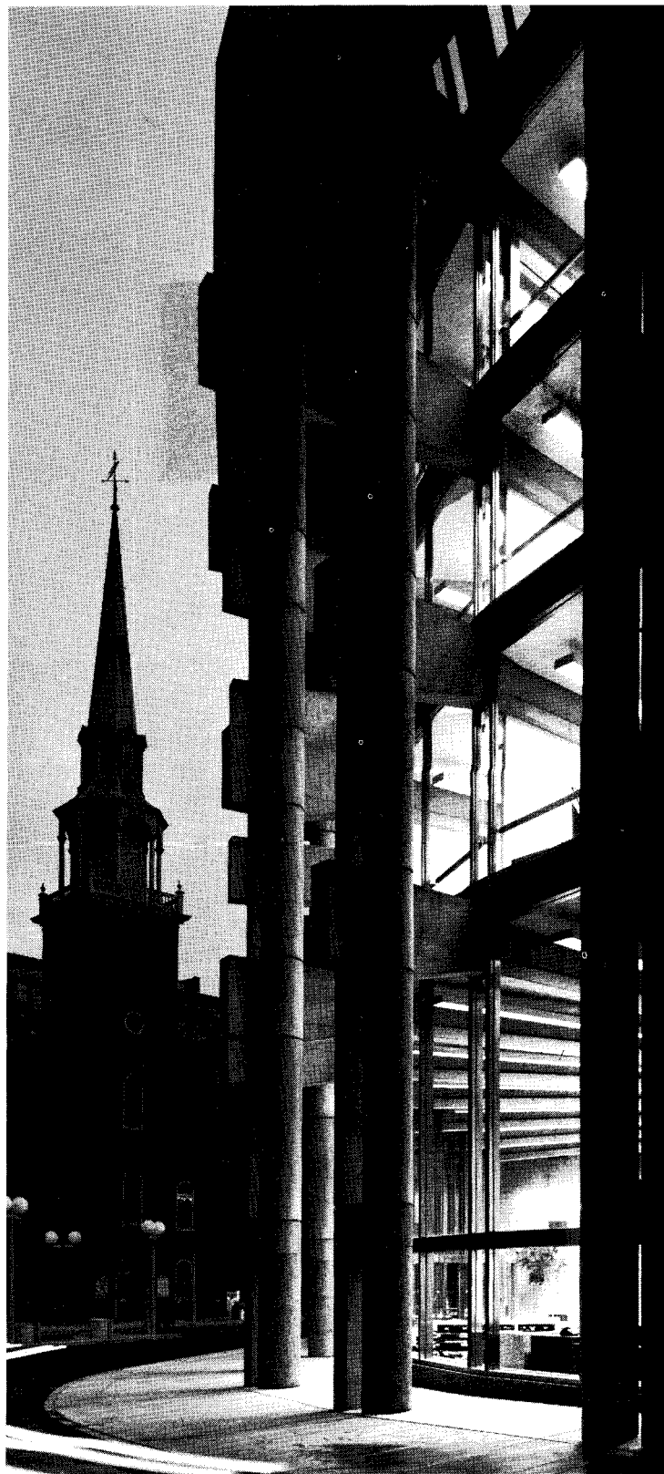
At the Boston Five Cents Savings Bank, cast-in-place columns, receiving post-tension beams, comprise a seven-ft.-wide, 65-ft.-high colonnade (above) which shelters pedestrians, protecting the north-oriented glass facade. The colonnade frames office views of such landmarks as Old South Meeting House (left and opposite). The spoke-like beams taper in depth from five to two-and-one-half feet, spanning a variable from 66 to 76 feet.
