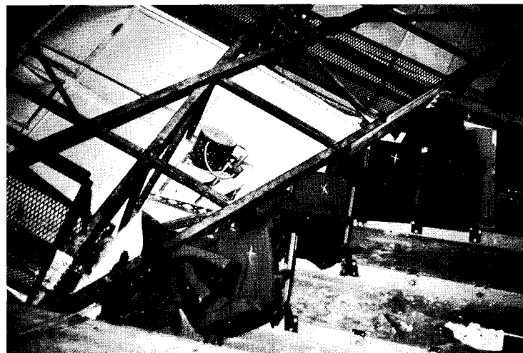
Part of the steel frame of aluminum clad ceiling now rests on the seats.
