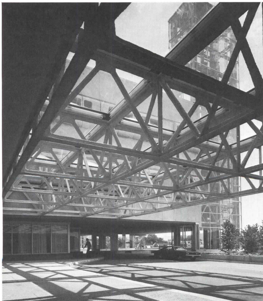
The canopy over the main entrance at McMaster (below) is an extension of the main trusses, 8 ft. 6 inches deep, that create the interstitial mechanical spaces of the building. Here they are light, airy, an appropriate introduction to the spaces inside.
