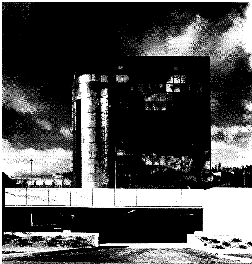
Copper molecularly bonded to stainless steel sheaths the cylindrical service core and street level columns, while gold-tinted reflective glass in a bronze anodized aluminum frame wraps tightly around the office block. The building sits on a reinforced concrete parking level that's been inserted into the 12-foot drop of the sloping site. On its roof a plaza was created, paved in native stone aggregate. Retaining and planter walls on the plaza have been sand-blasted for textural effect.
