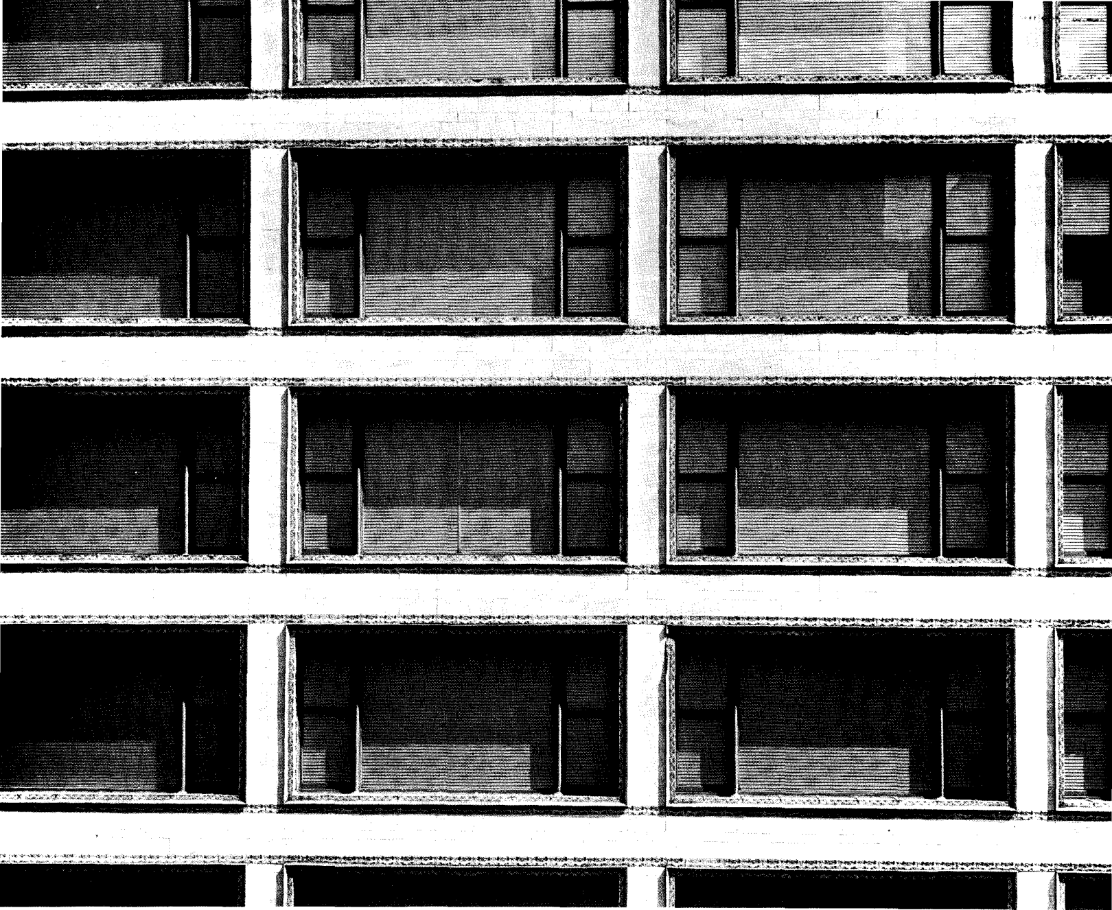
Carson Pierie Scott Building, Richard Sullivan, 1900.
