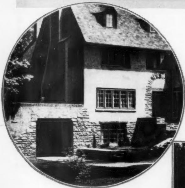
*The two-car garage above is built into the house, and the same heating and lighting system supplies dwelling and garage*
