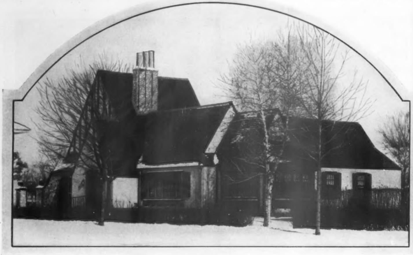
*If one needed proof of the heat-wasting quality of an uninsulated house here it is: the snow completely melted off the entire roof because of escaping heat*
