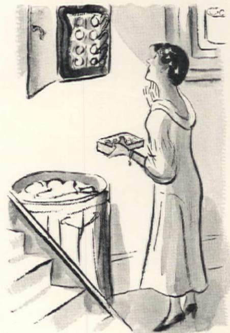
Replacing a "blown" fuse is an exceedingly simple operation provided you know which one of the fuses to change
