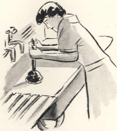
Frequent use of a "plumber's helper"—a stiff rubber cap with wooden handle—will keep the kitchen sink drain clear
