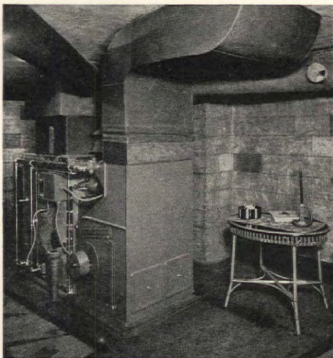
Here an air conditioning system used in connection with an oil burner has replaced an old-fashioned coal heating system and enabled the owner to make an attractive room of his basement. (Carrier-Lyle)
