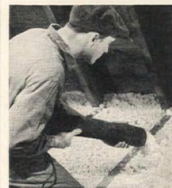
Blowing "rock wool" between attic joists. The empty spaces in the walls can also be filled easily by this method—blanketing the entire house.
