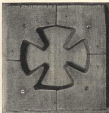
The moulding frame in position to pour the center cast of a two-color cement stepping stone
