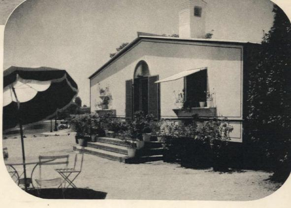
A MERICA'S first completely factory-built and portable house was recently announced in Los Angeles by Wallace Neff, noted California architect. Finished in the uttermost detail, and as thoughtfully furnished, even to flower-filled vases and framed prints for the walls, this unusual home was put on a trailer at the factory and quickly transported to a prominent site on fashionable Wilshire Boulevard where it was set in place and was ready for all to see in a few hours.
