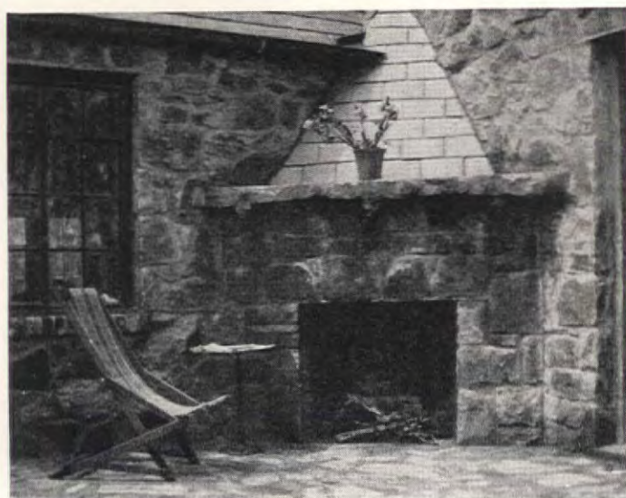
A corner fireplace just outside the dining-room door on an uncovered terrace creates a center around which to gather for after-dinner coffee. For other outdoor fireplace ideas see page 35
