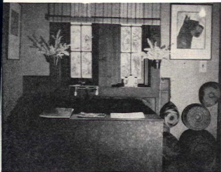
Corner of the dog room showing concealed wash tubs. The top is removable when the tubs are to be used. It is so arranged that it can be turned over and the under side used when stripping and brushing is done on top of it
