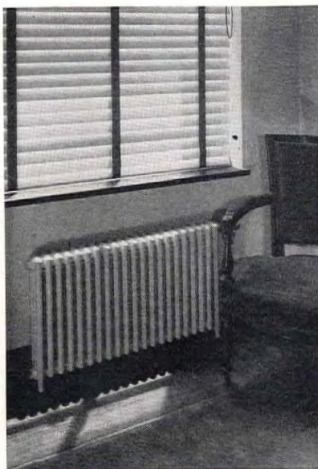
so little space that the supply lines had to be moved closer to the wall. And, at right, side columns and a top conceal fittings, giving a modern appearance. American Radiator
