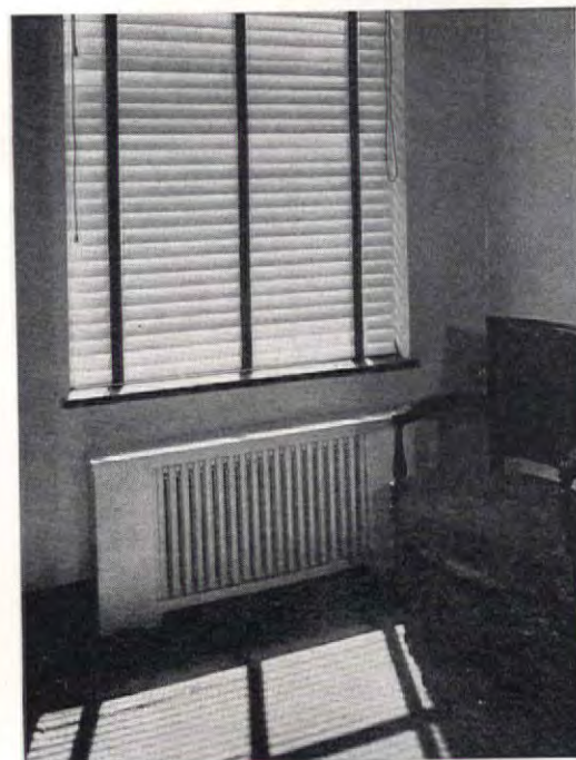
Top illustrations: What a vast improvement to the appearance of a room as well as being a space saver is the newer, more compact type of radiator that may be recessed in a wall. Burnham Boiler
