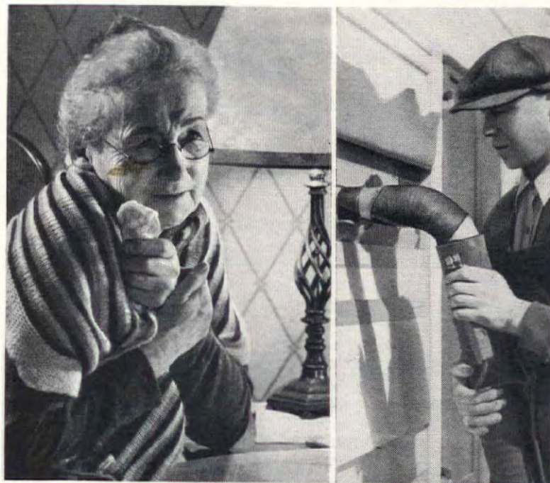
BY BLOWING J-M ROCK WOOL between attic floor joists and into hollow walls, this man puts an end to cold, draughty rooms.
