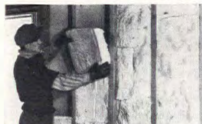
● J-M Rock Wool Insulation saves fuel. In "bats," as above, or blown into hollow walls.
