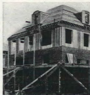
House construction of Gypsum lumber, a product of the Rockwood Corp. Above, laying floor units for a new house
