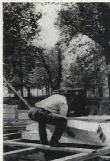
House construction of Gypsum lumber, a product of the Rockwood Corp. Above, laying floor units for a new house
