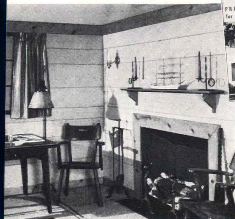
Unused space in the basement can become a cheerful extra living room at low cost. Johns-Manville Insulating Board for the ceiling and Johns-Manville Asbestos Flexboard for the walls do the trick effectively, as shown above.
