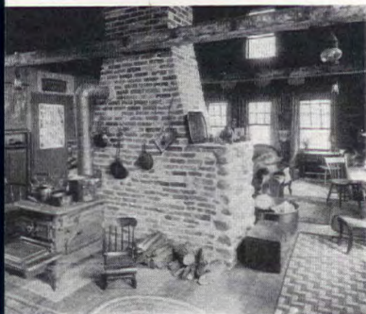
The central chimney with fireplace on one side and kitchen range on other side
