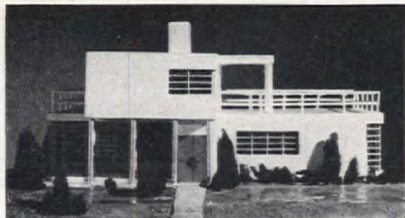
This copper house is now being built in Virginia, just outside Washington, D. C. Rooms can be rearranged like those in office buildings, since the partitions carry no load. Copper Houses, Inc.
