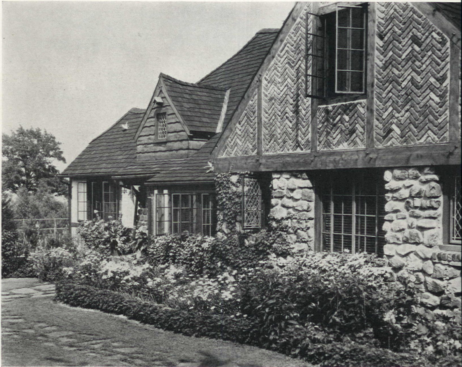
The foundation of the house is beautifully banked with hardy perennials. The house itself is but an edifice within a rock garden
