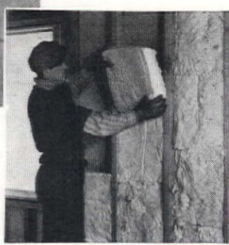
● J-M Rock Wool Insulation keeps rooms cool in summer, shuts out cold in winter. In "bats," as above, for new construction, or blown into hollow walls of present houses.
