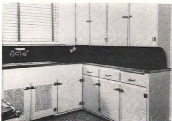
The kitchen has a new sink and black linoleum drain-board bound with bright chromium strips
