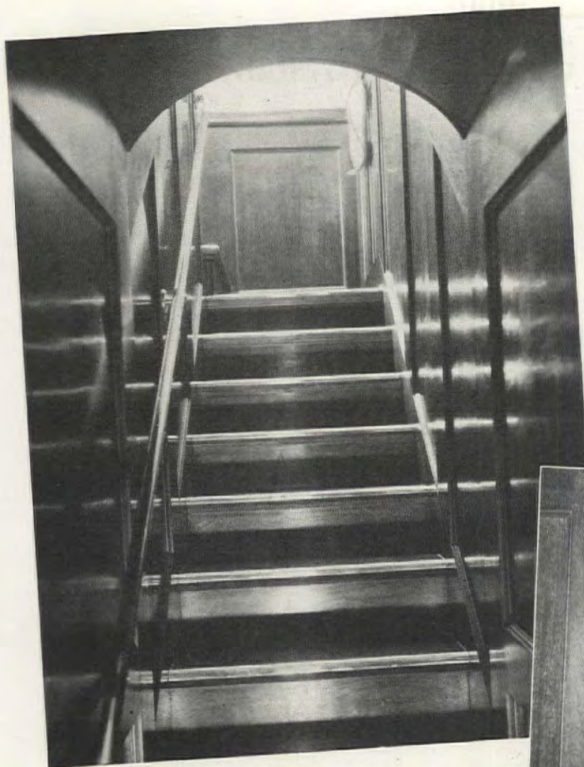
The only structural change was that of narrowing up the stairwell to resemble more closely a ship's companionway
