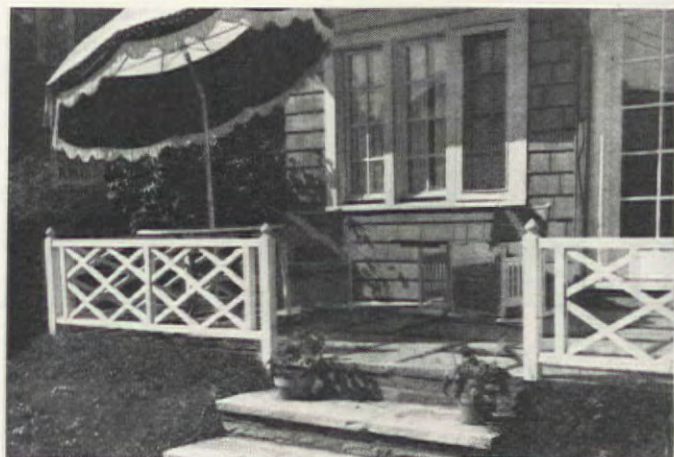
A view of the new terrace showing the paving—flagstones in odd shapes with bent lawn grass growing between stone steps. The windows shown are in the sunroom
