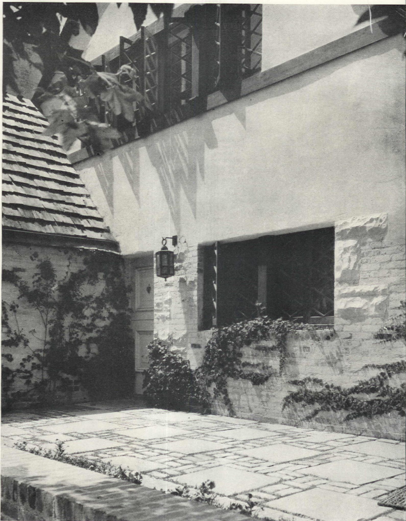
Old brick and cast stone blocks harmonize to make an inviting entrance to the plaster and brick veneer house. The use of bricks painted white, with plaster above the windows, has the effect of keeping the house low, suggesting the English cottage tradition
