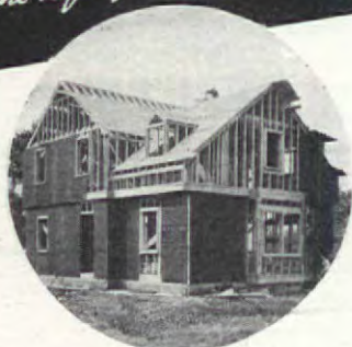
Celotex outside the framework replaces ordinary sheathing—gives strong, wind-tight walls
