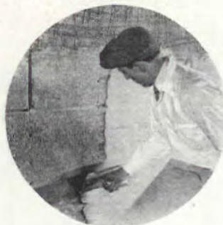
Celotex inside the framework eliminates other lath—gives stronger, smoother plaster walls
