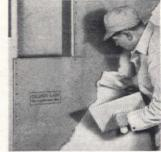
How plaster is applied direct to Celotex, ng stronger walls permanently p tected from lath marks
