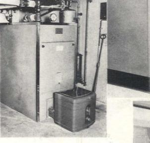
Iron Fireman "Coal Flow" stoker installed in American Radiator Co. stoker-boiler
