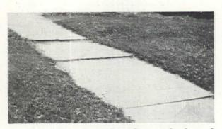
Water unable to escape through a poorly drained lawn area may freeze and throw flags out of line
