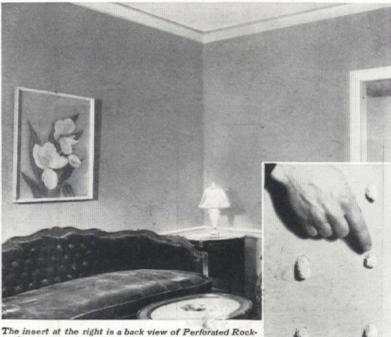
The insert at the right is a back view of Perforated Rocklath<sup>\*</sup>, showing how Red Top Plaster penetrates the perforations and anchors to the lath, providing an extra grip, in addition to the natural bond of plaster to the lath.
