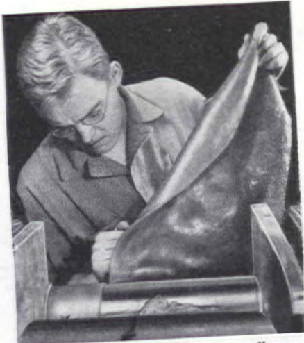
2 Our Own Rubber Mill is busy all year with samples and experimental batches. This sheet of pure rubber will be a new-type Plymouth body mounting.
