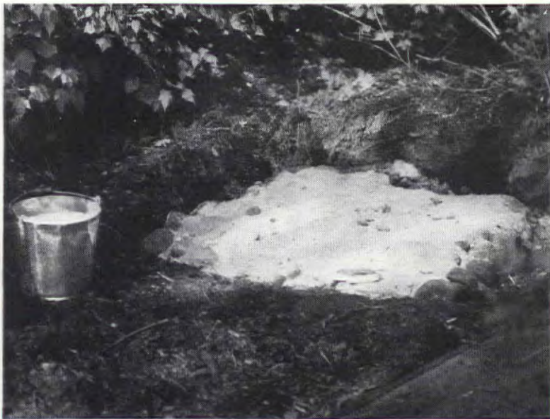
Figure 1. A layer of small, flat stones was covered with sand
