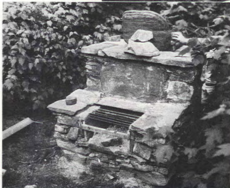
Figure 6. A wind shelf was built in to prevent back drafts
