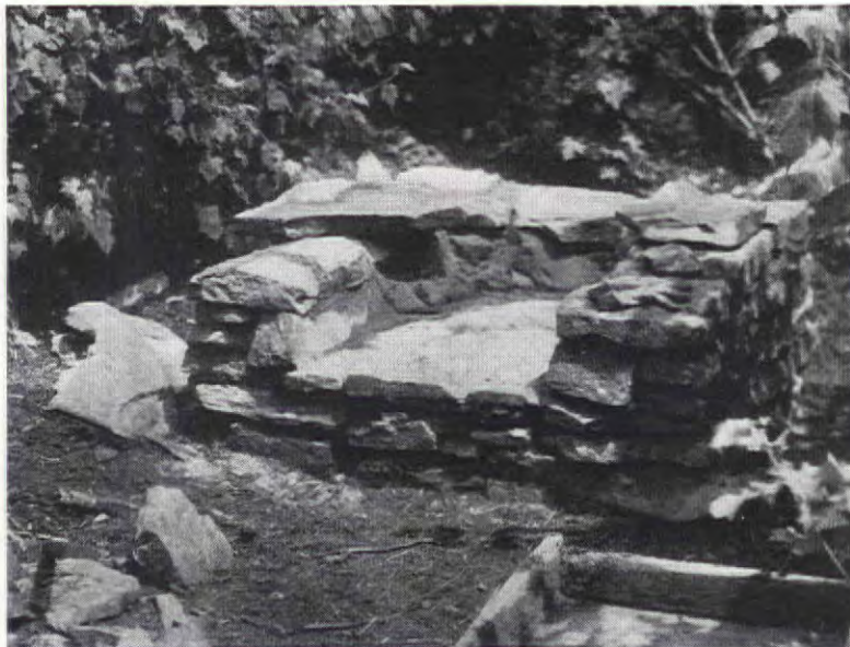
Figure 2. Back and side walls were built up to about eight inches
