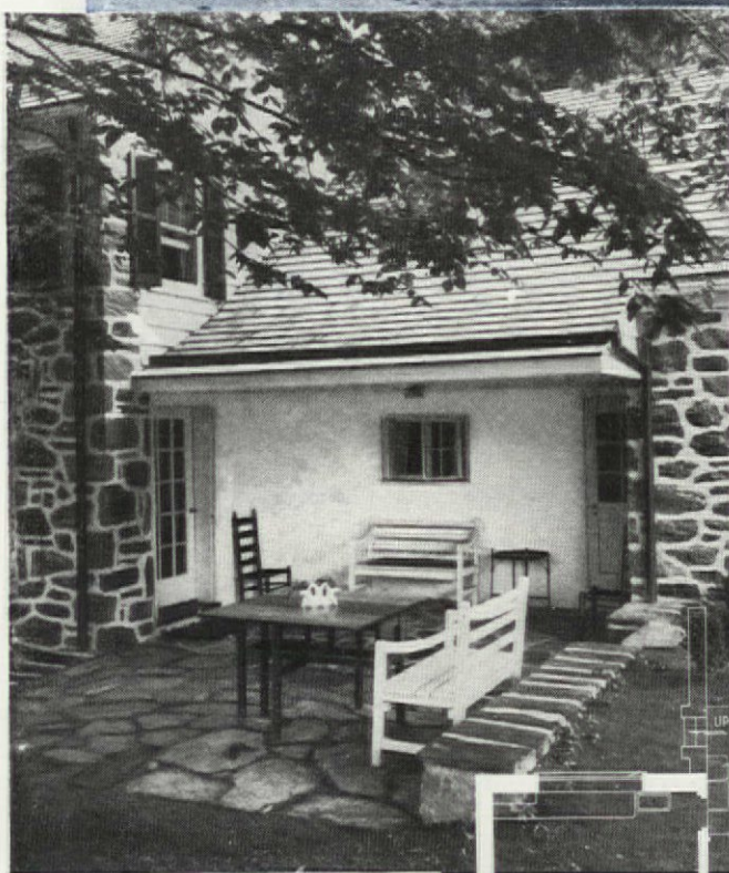
For outdoor dining convenience, the rear terrace is reached by kitchen and dining room. It is recessed, roofed, and stone-paved
