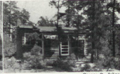
Home of Ralph L. Bancroft, Browns Mills, New Jersey
