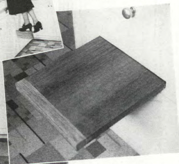
Left, detail of draw-step shown in use above. It is sixteen inches up from the floor. Above, another type of disappearing draw-step
