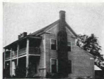
Gable removed and columns boxed in
