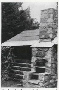
Outdoor fireplace with damper control and pully wire which opens oven door
